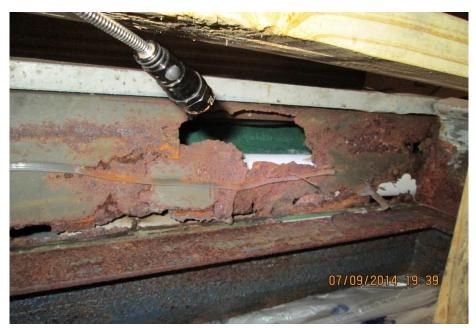
Figure 2: South Wall Corrosion of Intake Louver Framing
