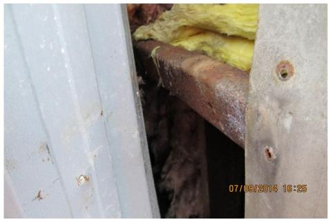
Figure 3: East Wall Corrosion of Lower Girt
