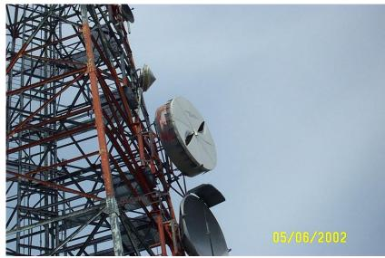
Figure 3: Heavily Damaged Radome
