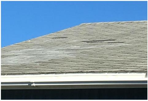
Figure 3: Roof – Shingles lifting and deformed
