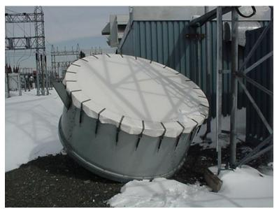
Figure 1: Microwave Antenna with Radome
