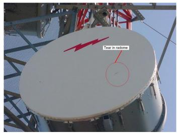
Figure 2: Tear in Radome
