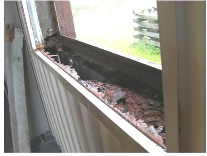
Figure 1: South Wall Corrosion of Horizontal Girt
