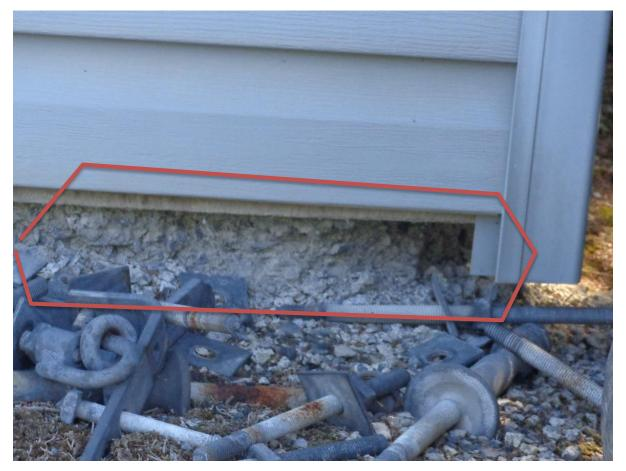
Figure 4: Deteriorated Concrete Slab under the Storage Shed walls
